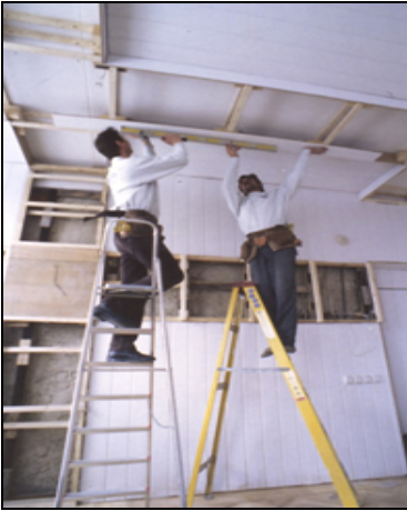
Installing a suspended ceiling
